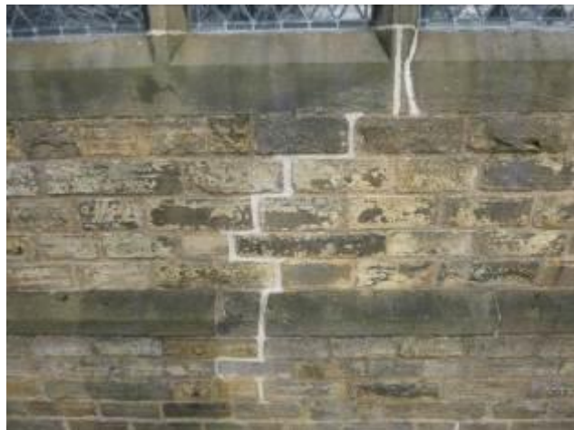
Repaired stepped crack to St. Mark's Church
